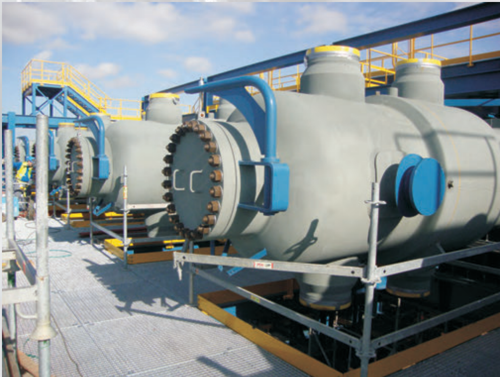
Battery of shell & tube heat exchangers in solar power plant
