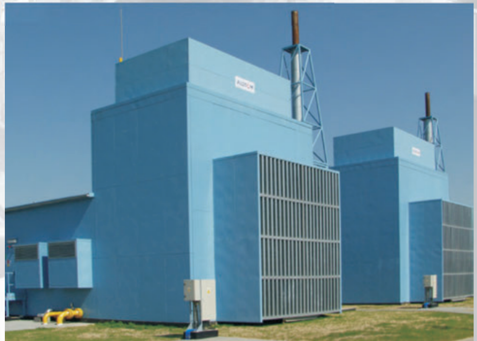
Natural gas air coolers in soundproof housing
