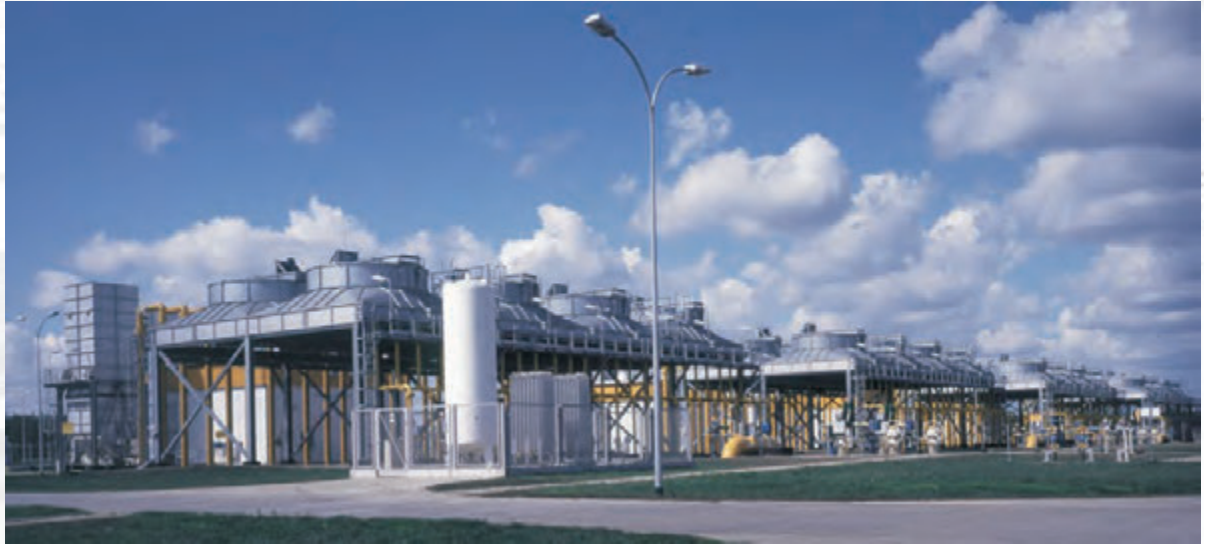
Battery of natural gas air coolers
