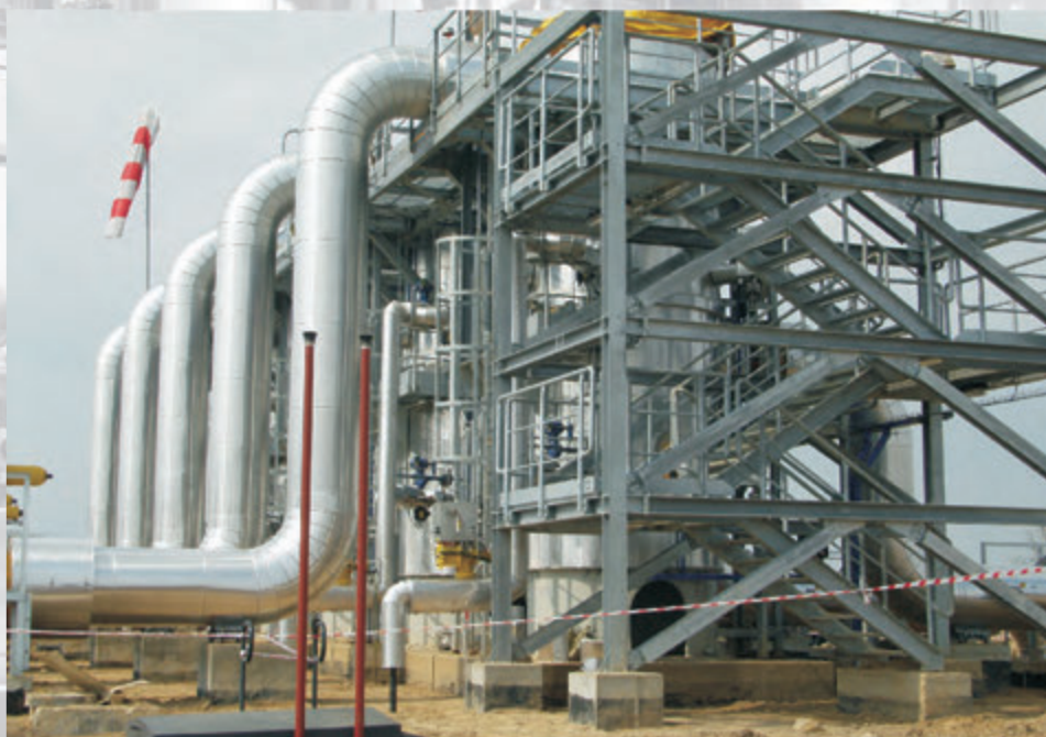
Gas filters station in compressor gas station
