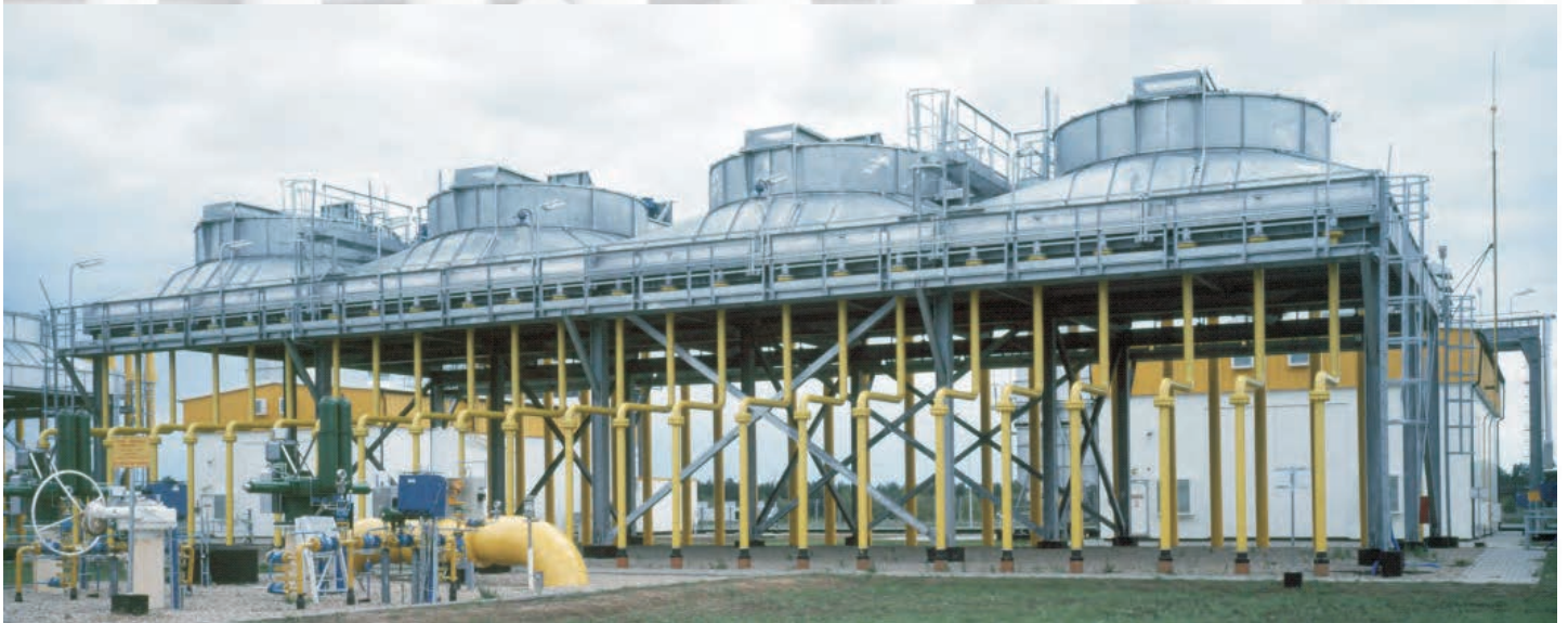
Automatically controlled louvers installed in air cooler
