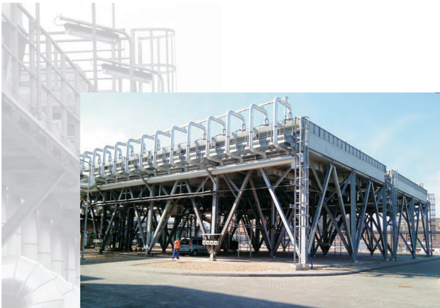
Glycol air cooler in thermal-electric power station
