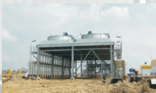
Battery of natural gas air coolers
