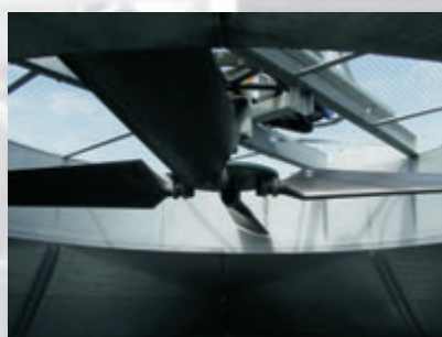
Fans installed in natural gas air coolers
