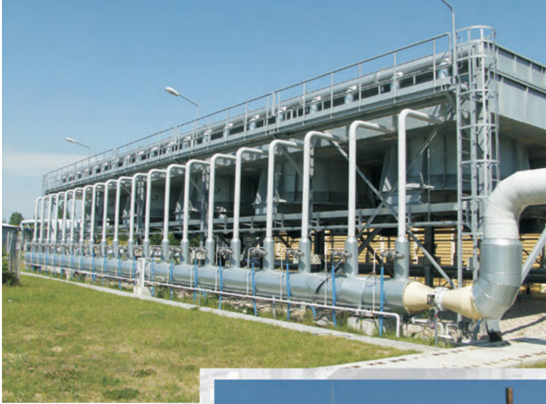
Water air cooler in power station
