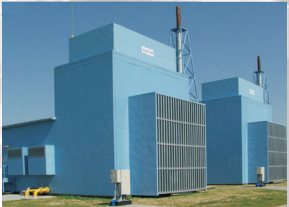
Natural gas air coolers in soundproof housing
