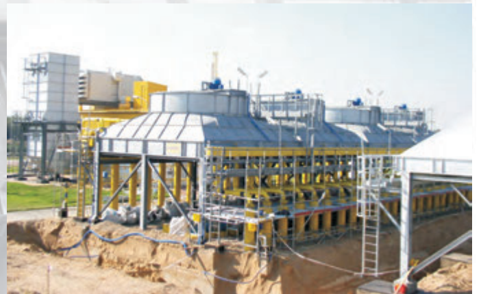
Collectors in compressor gas station
