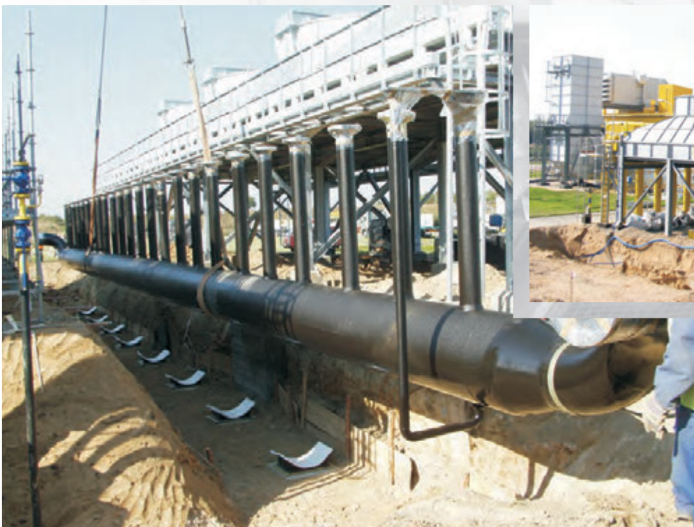
Collectors in compressor gas station
