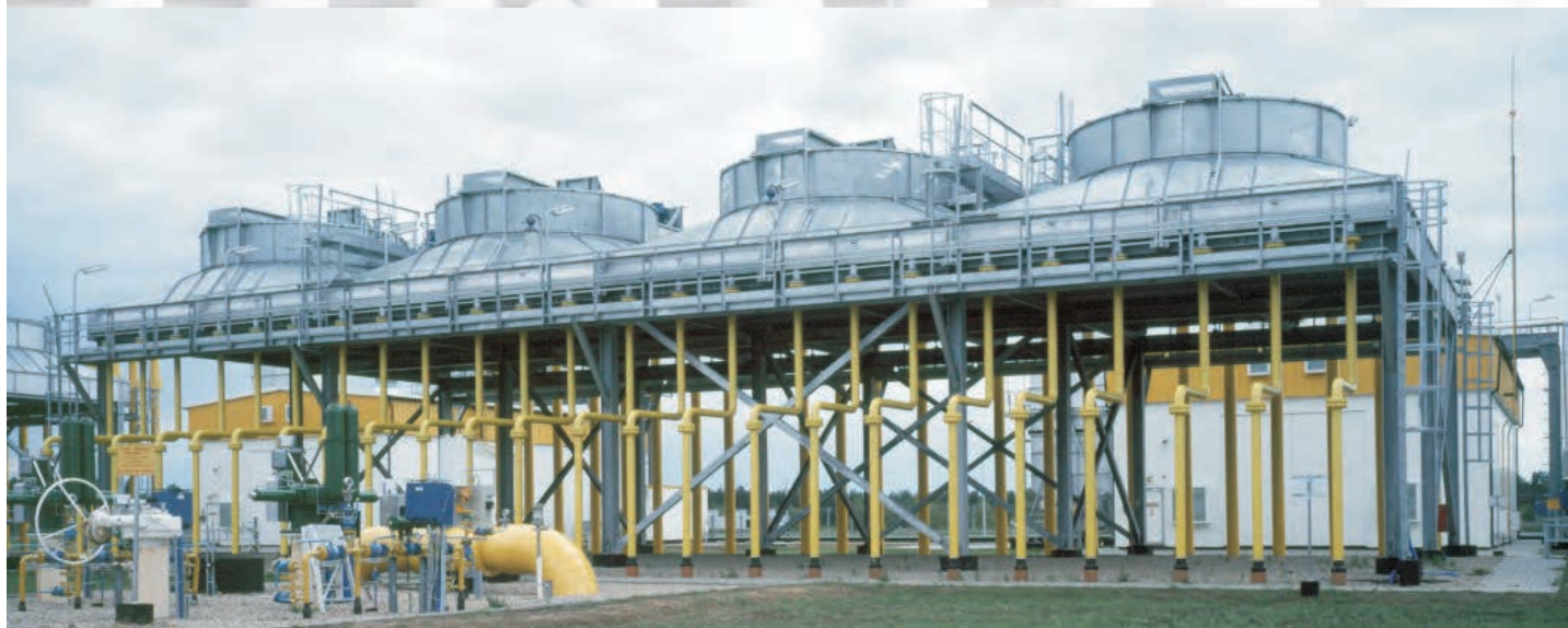
Automatically controlled louvers installed in air cooler
