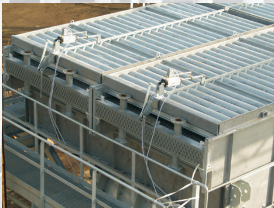
Automatically controlled louvers installed in air cooler
