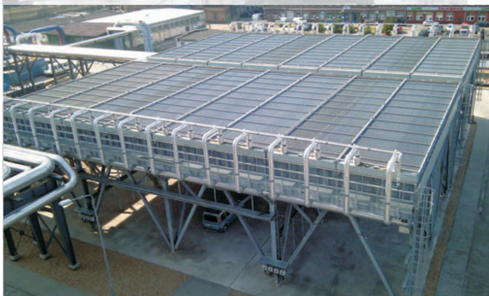
Glycol air cooler in thermal-electric power station
