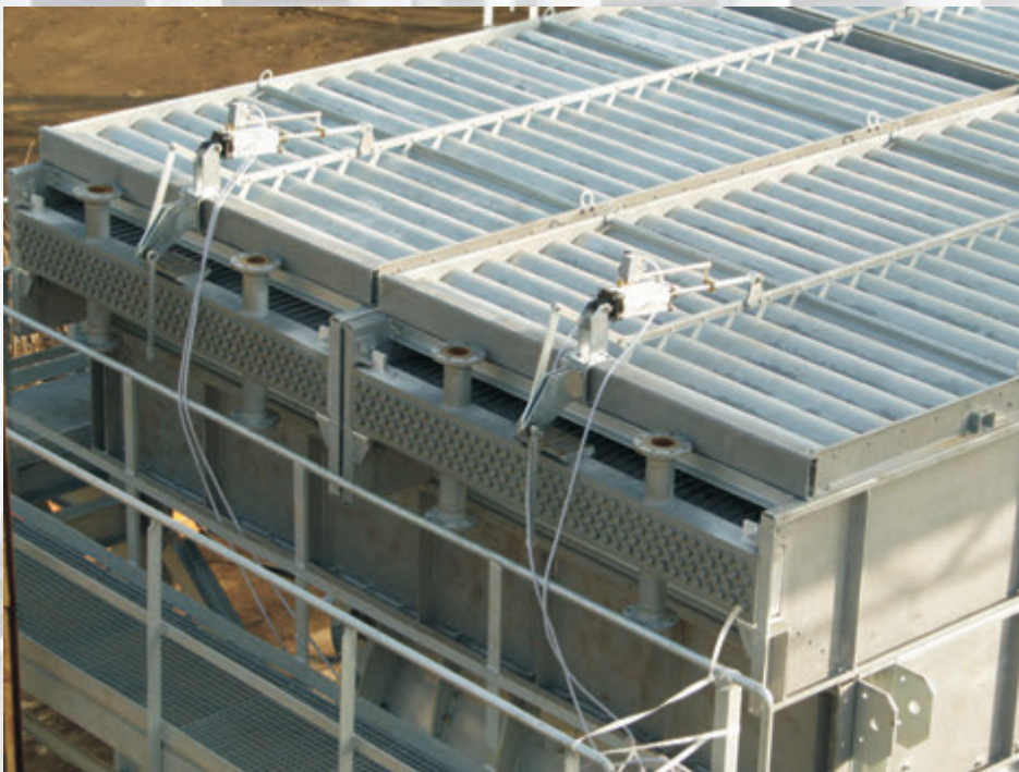
Automatically controlled louvers installed in air cooler
