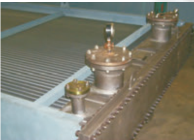
Water pressure test of tube bundle
