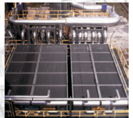
Air cooler installed in chemical synthesis plant
