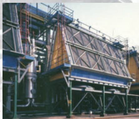
Air cooler with tube bundles in roof arrangement
