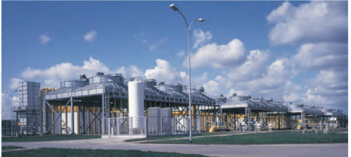
Battery of natural gas air coolers
