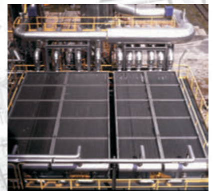
Air cooler installed in chemical synthesis plant
