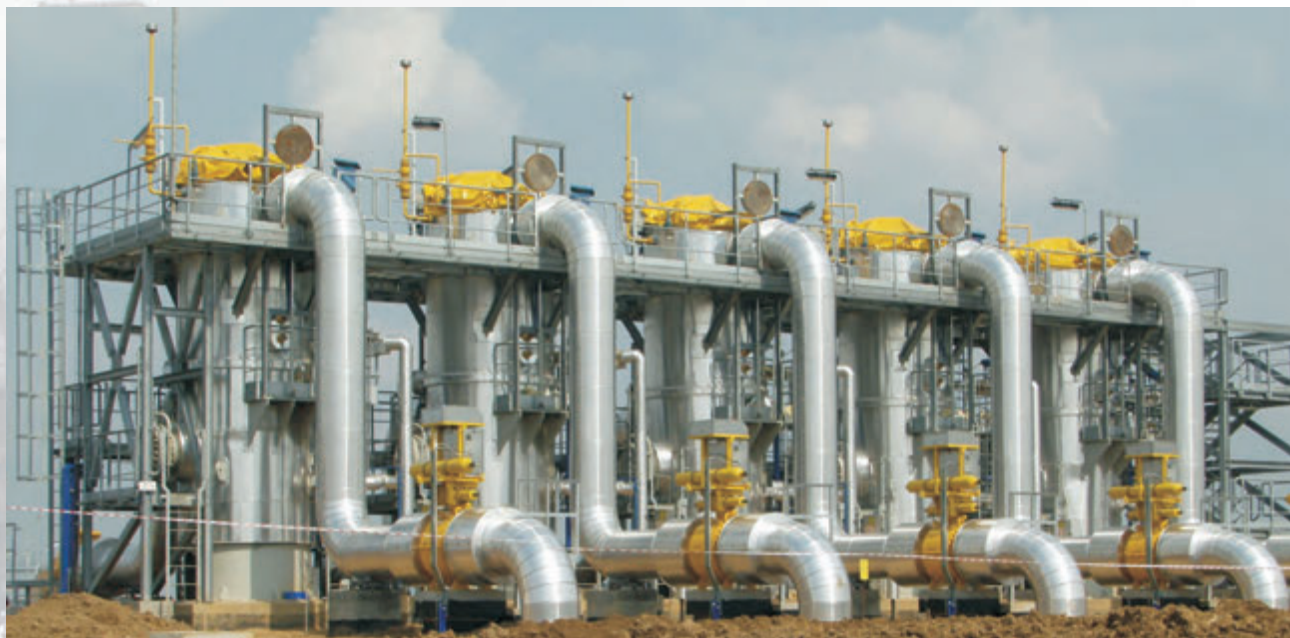
Gas filters station in compressor gas station
