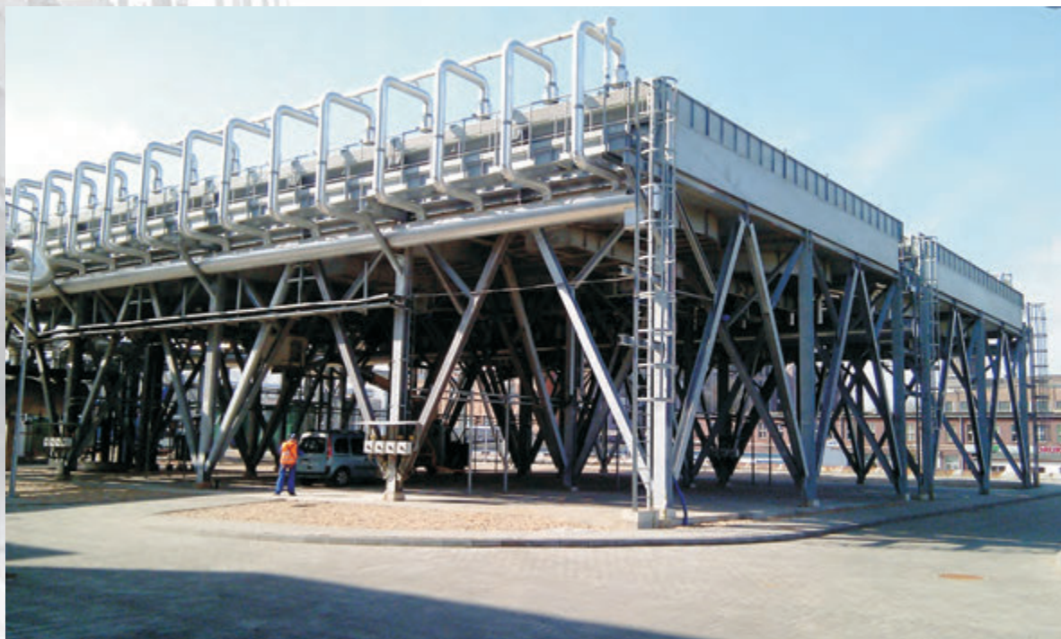
Glycol air cooler in thermal-electric power station
