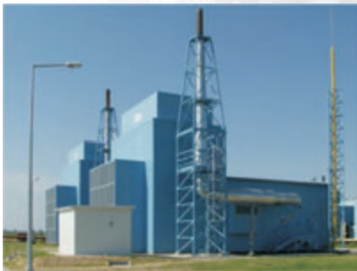
Natural gas air coolers in soundproof housing
